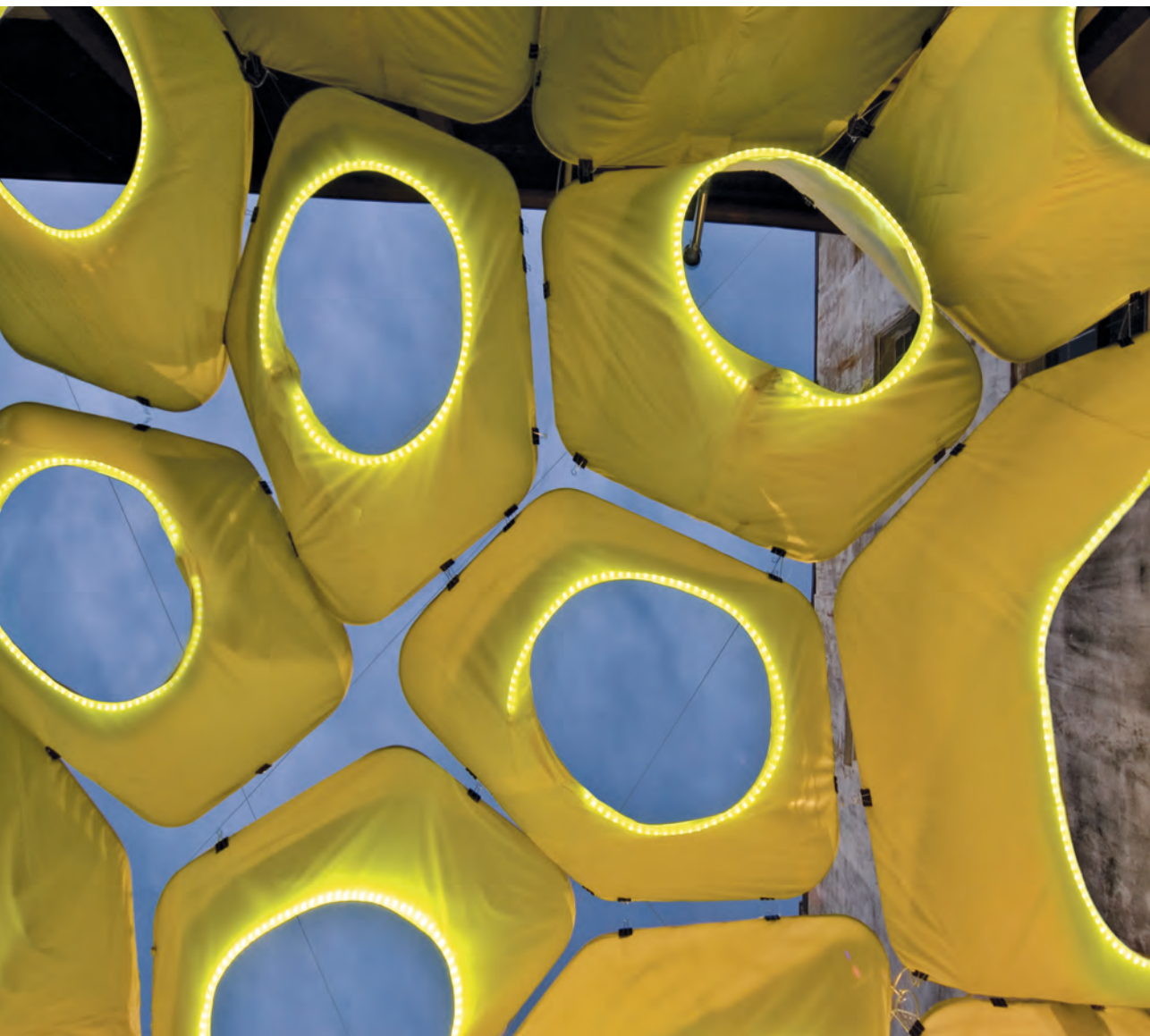
Höweler + Yoon Architecture, LLP, Hover , New Orleans, Louisiana, USA, 2007, view from below. LED lighting embedded in the canopy fabric is powered by a solar-charged battery. © Höweler + Yoon Architecture, LLP.
